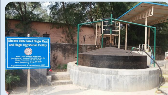
Biogas production, enrichment and bottling facility at BDTC IIT Delhi
